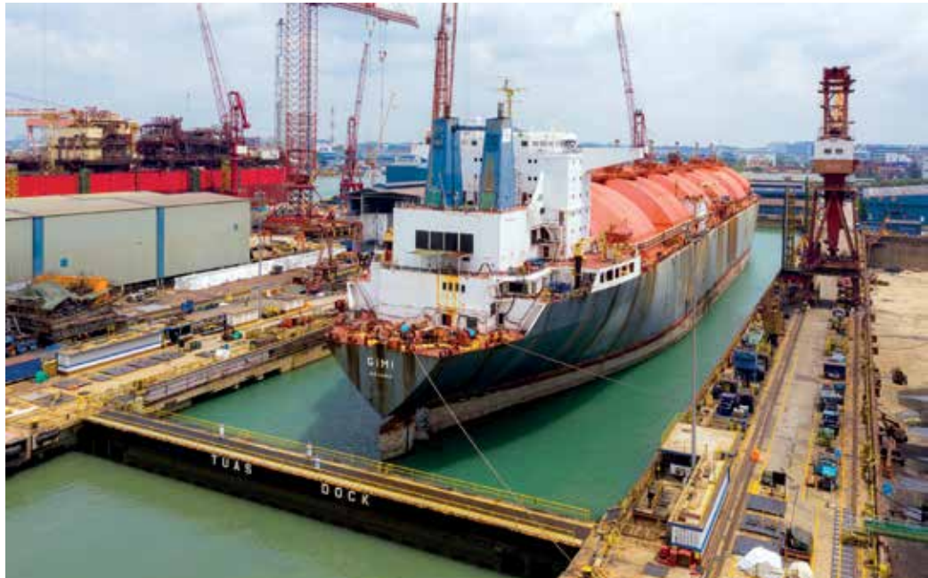
The Gimi is already in Keppel Shipyard which has completed the early works relating to design verification, engineering and some physical assessment works on the vessel
