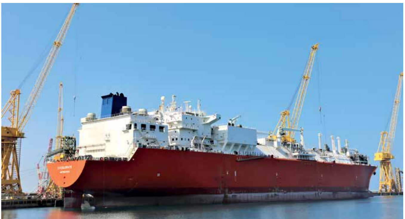
The 138,000m 3 Excelebrate is the first FSRU project for N-KOM
